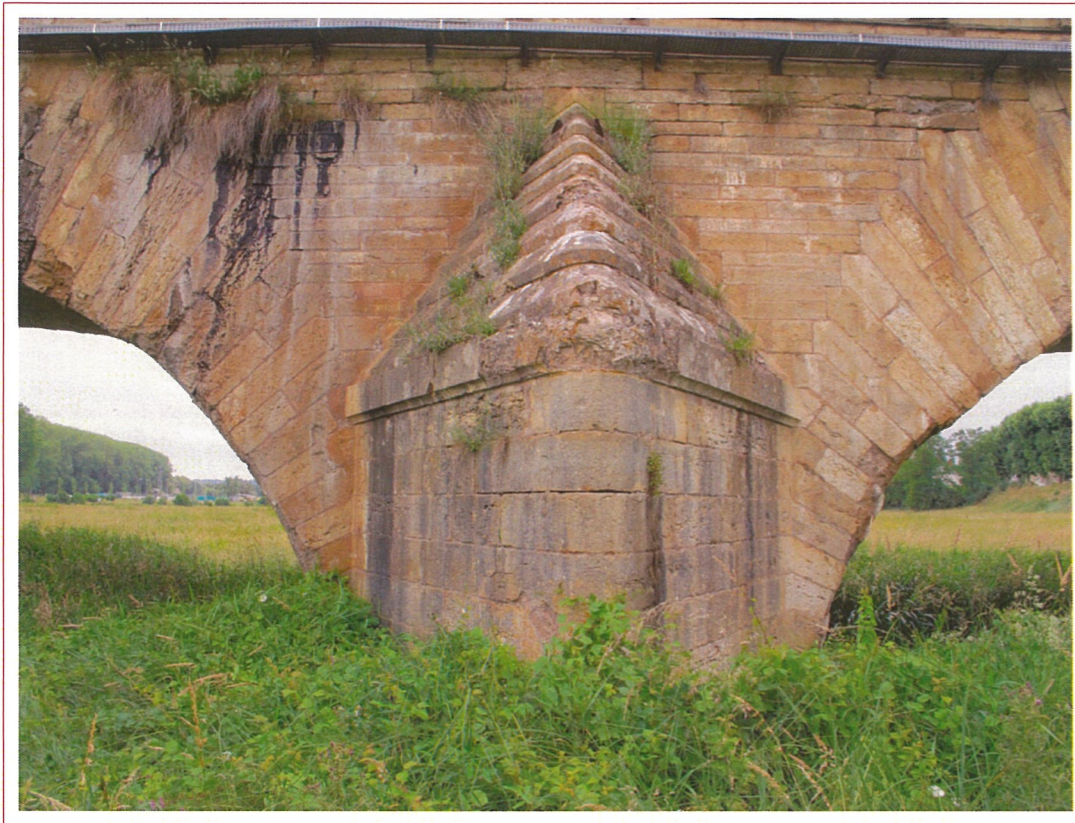
Avant bec Pile 6 Disjointoiement -Photo 38-
